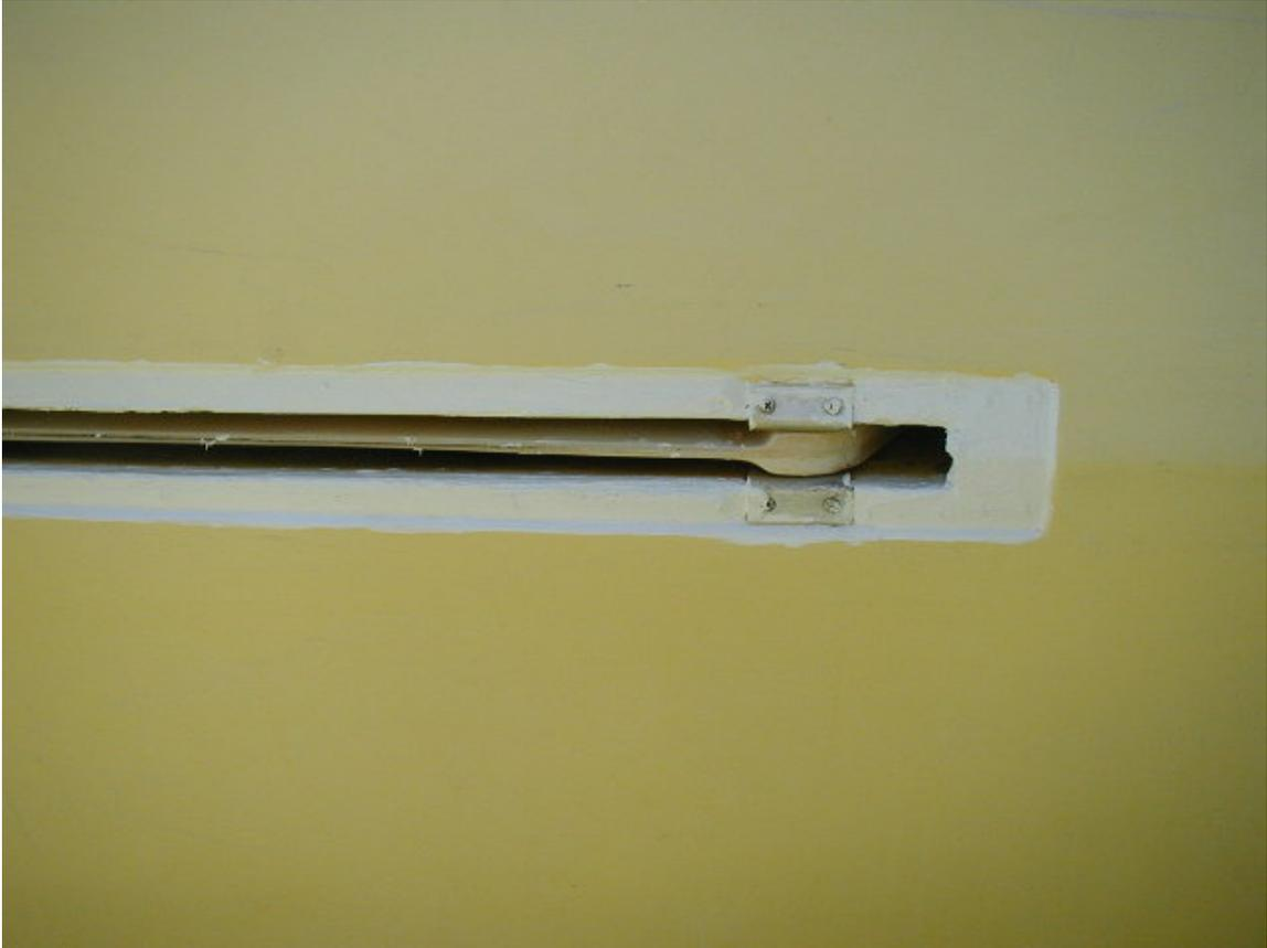
This is the slot prepped and ready to have the gasket material glued on. I decided to eliminate the aluminum strips, so I filled in the holes with Marine-Tex. It is a good idea to fill the old screw holes even if you plan to reuse the aluminum strips because this can be an area of leaks. Of course, if you fill the holes with Marine-Tex, or anything else that solidifies once it dries, the holes for the screws must be predrilled.
