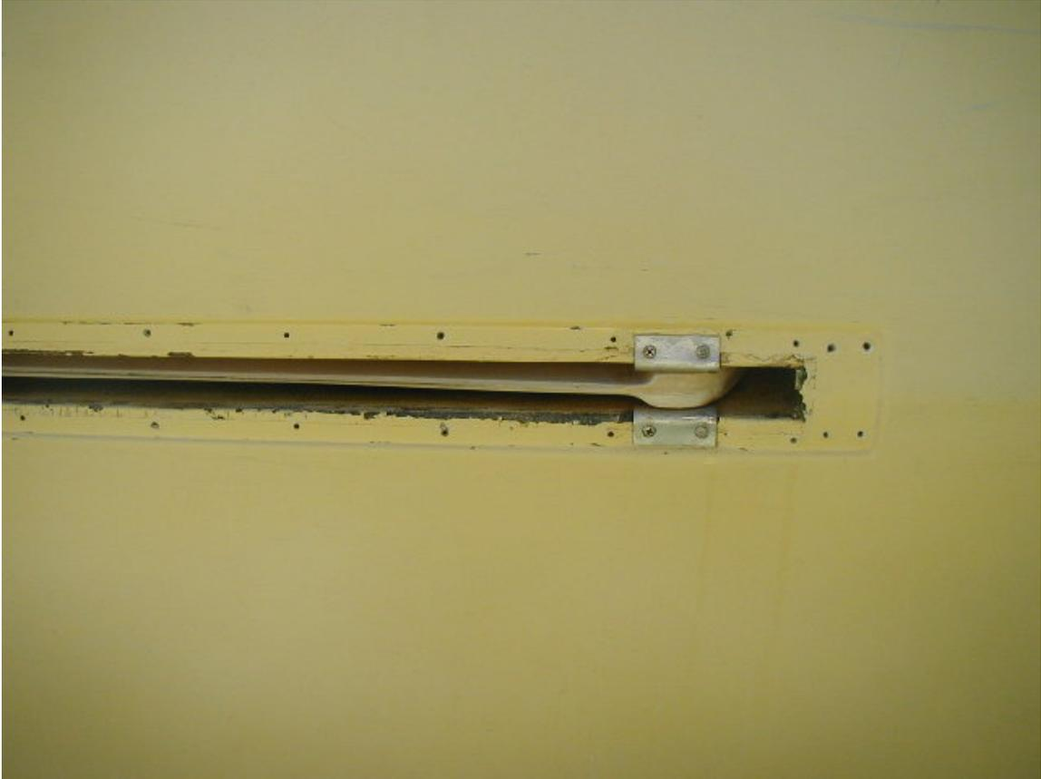
This is a picture of the slot with the old gasket removed, and all of the old glue cleaned off. The first thing that you need to do is remove the aluminum strips. They are attached with wood screws. Once they are removed you can pull off the old gasket and clean off all of the old glue.
